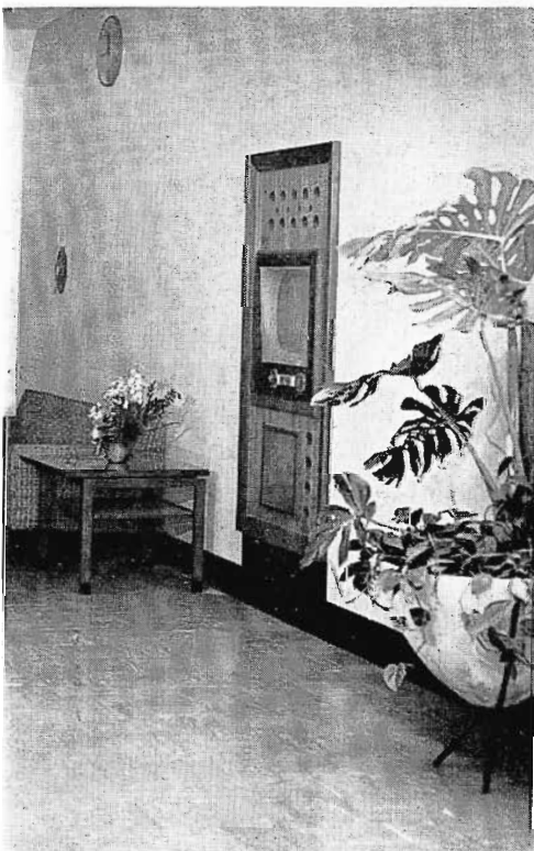
FIG. 31. House monitor located in main lobby. Receiver is mounted on runners which permit chassis to slide out for servicing.
