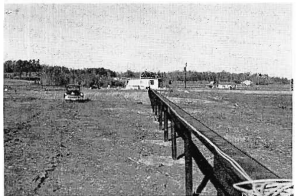
FIG. 8. Creosote-treated raceway from the WCBI transmitter house to tower #3 shown in this view carries the transmission line, power cable, supervisory wires, sampling lines and communication wires between the towers and the transmitter house.
